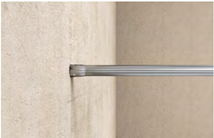
Hohlbohren in Betonwand
