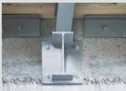
Fixing of steel beams, consoles and handrails
