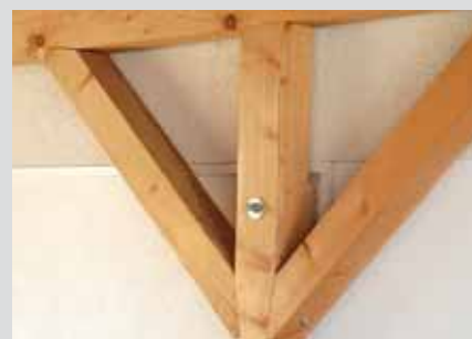
Fixing of timber structures
